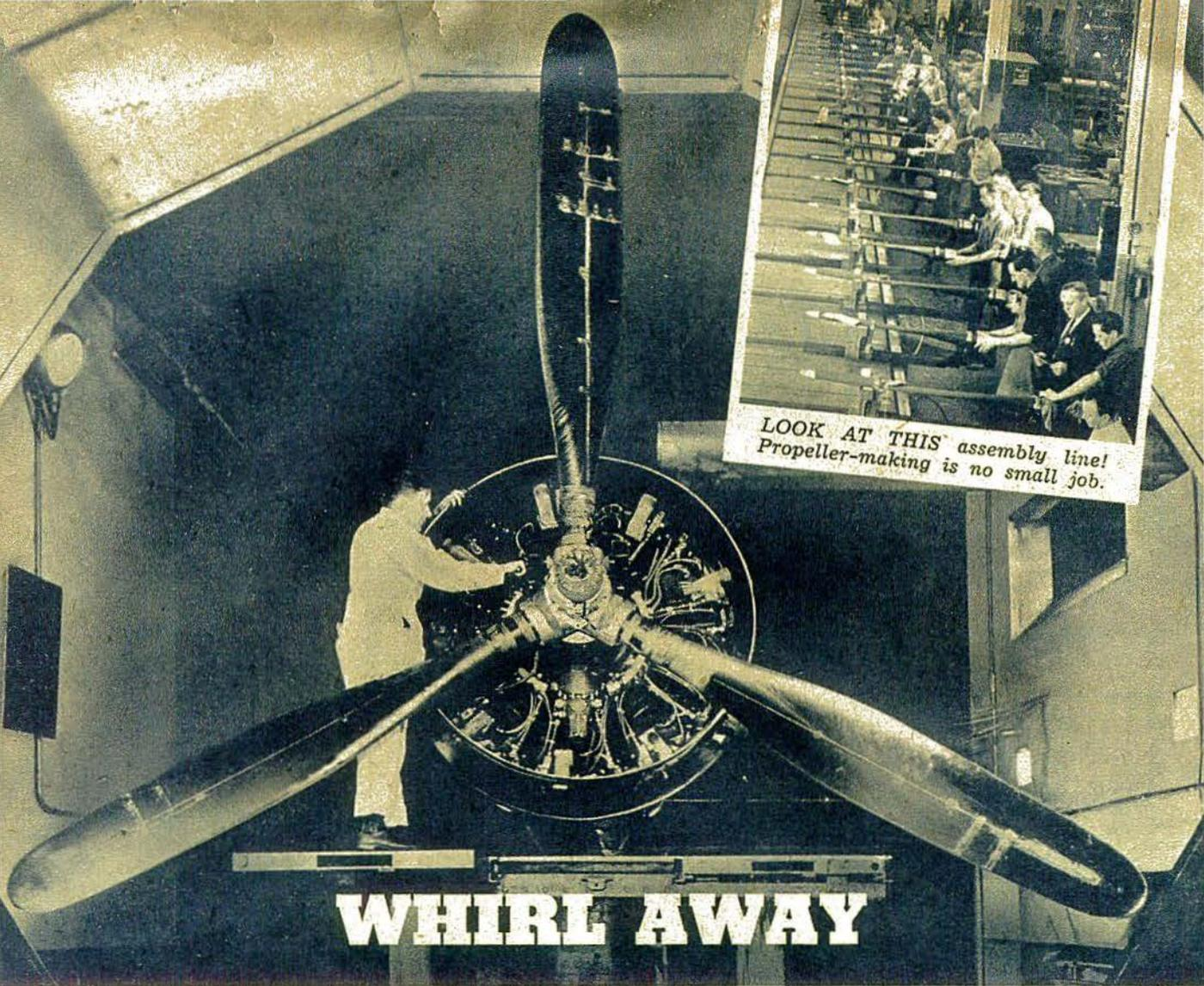
*GIANT PROPELLER DESIGNED for bombers and troop transports which must brave the stratosphere. This picture shows the world's very largest propeller undergoing stringent tests in the testing chamber.*
